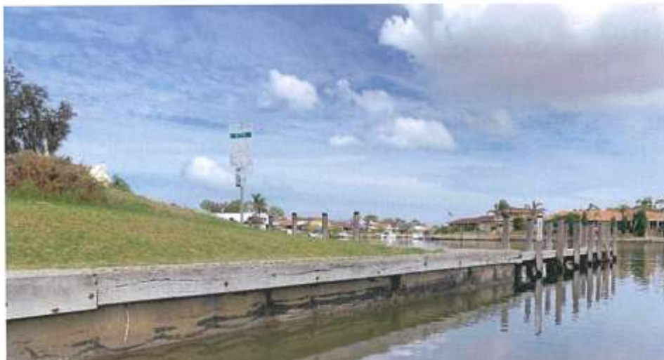
Figure 1 Timber Boards Attached to the Top of Wall
